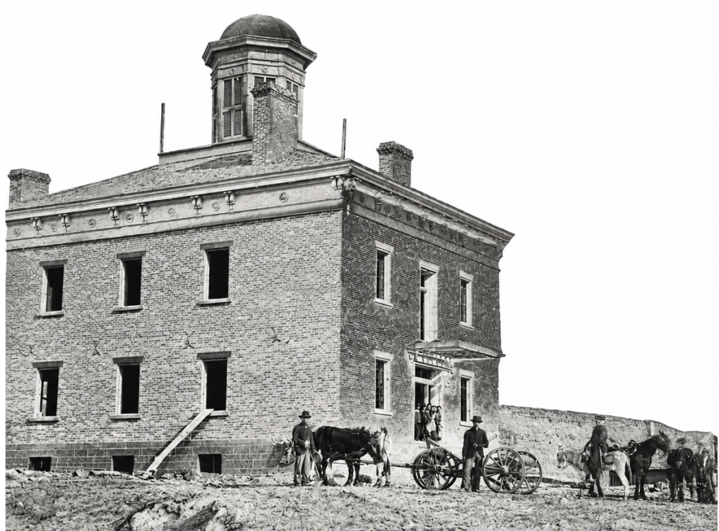
Figure 5 St. George Courthouse. Still standing today, 2026. The corners and walls are precise and straight
