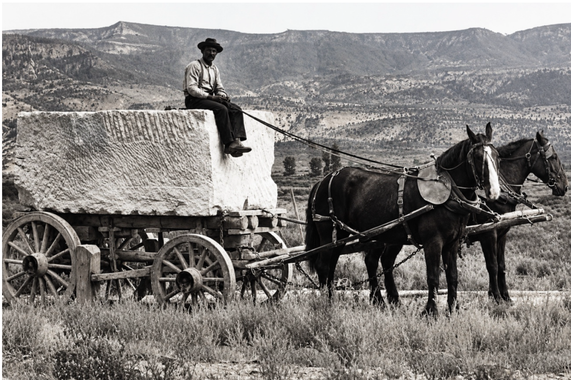
Figure 7 Building with rock was the dream. The rock masons of Utah made it happen.
